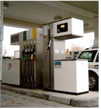
Natural gas filling stations
